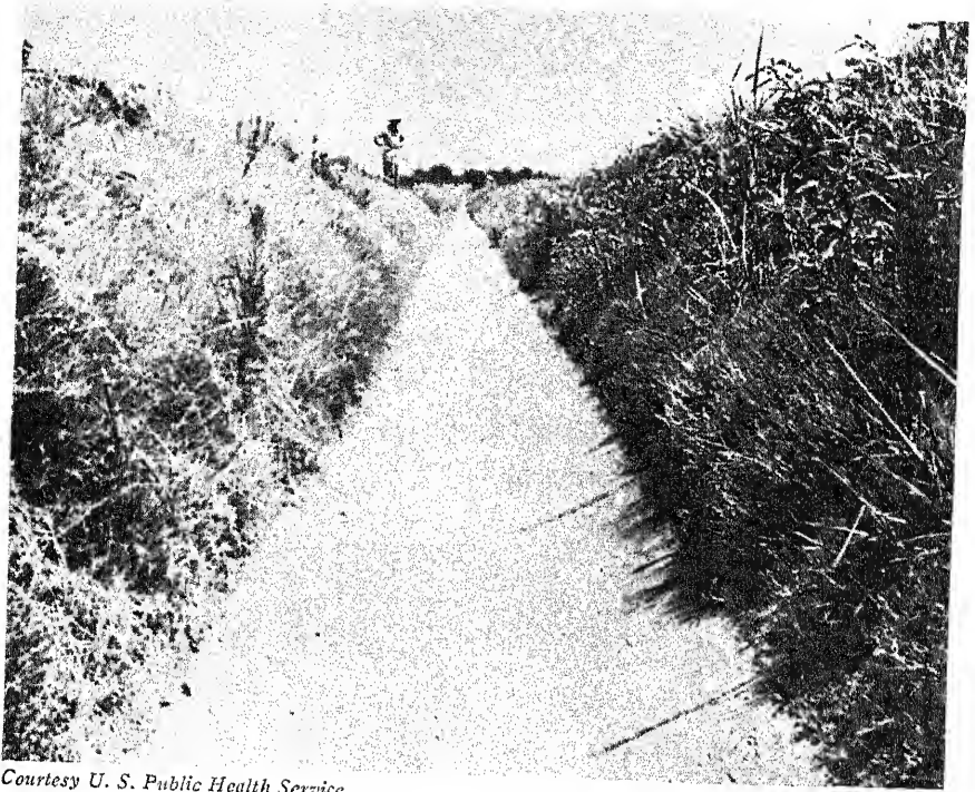
Figure 32. Precast concrete invert used as drain ditch bottom lining
